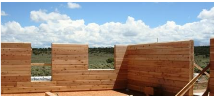
Window & door openings (with measuring spacer)
