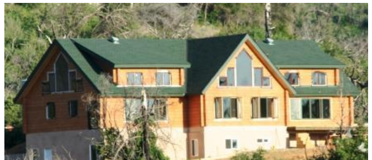
This S California log home nearing completion has active solar and wind power.
